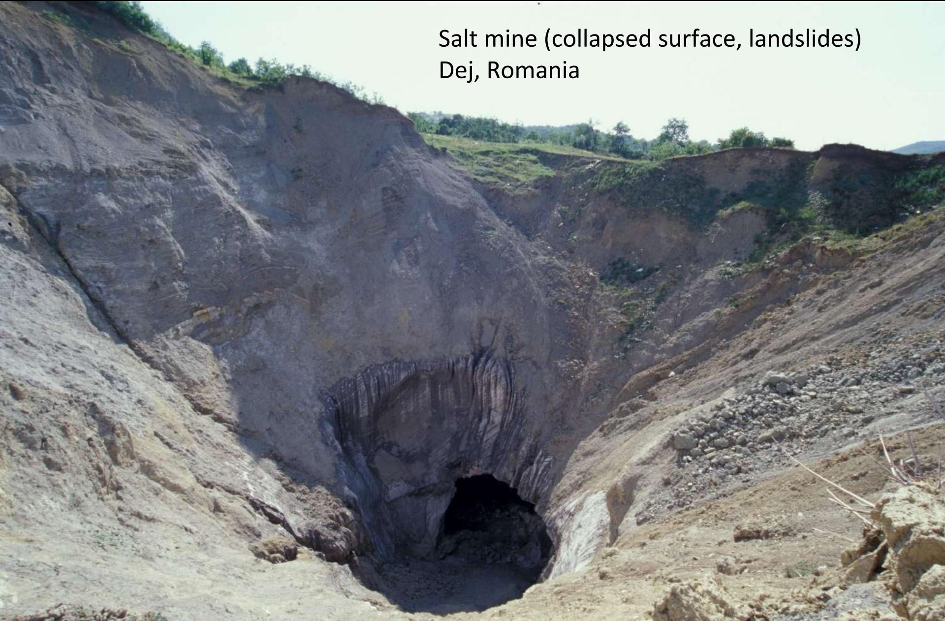
Salt mine (collapsed surface, landslides, old mining channel)
